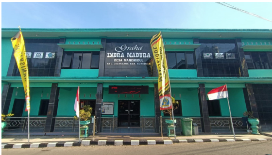
Figure 16. Manis Kidul Village Office as Kampung Nagara (Source: Documentation Eko Budi Prasetyo, 2022)
