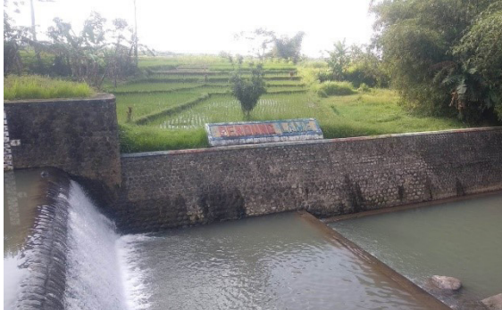
Figure 12. Lame Dam used to irrigate residents' rice fields (Source: Documentation Eko Budi Prasetyo 2022)
