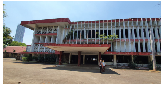
Fig. 2. The Facade of The Building (Source: Survey Result of team in 2020)
